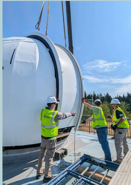
South arch being lowered into the dome.
