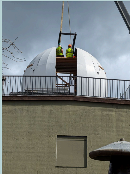
North arch being lowered into position.
