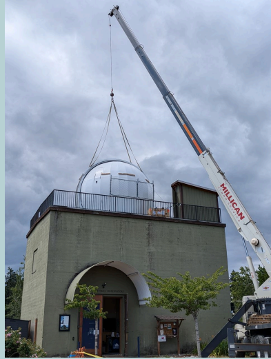
Shutter being positioned on the arches.
