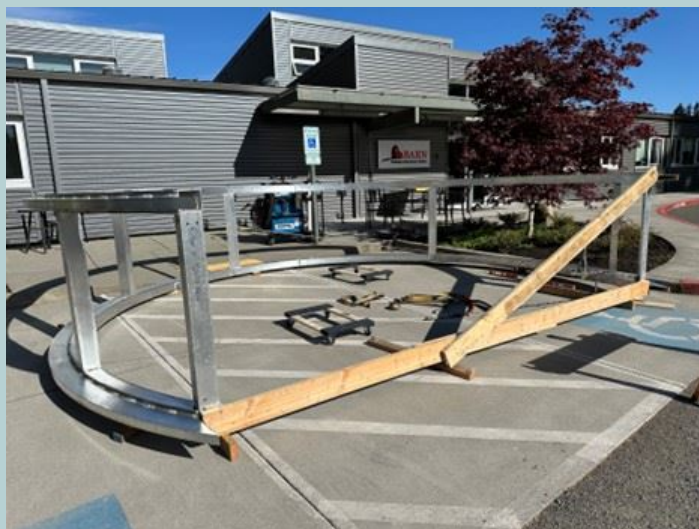
The arch assembly on it's side at BARN.
