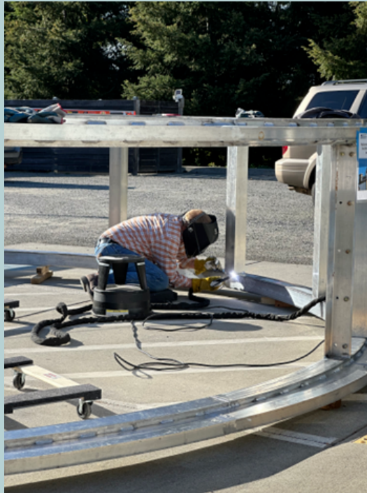
Here is Patrick Clanton welding the assembly.
