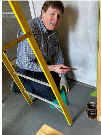
Dan Schlesener applying some stain to the woodwork.
