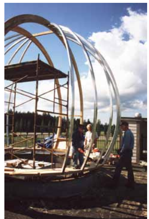
Volunteers build the dome.
