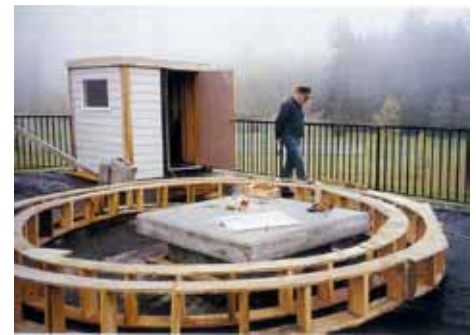
The foundation for the Ritchie Telescope Dome.
