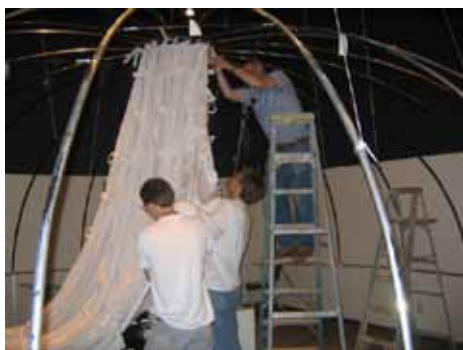
Hanging the domed planetarium screen.
