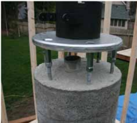
Close up of top of pier showing foundation bolts and conduit
