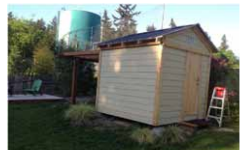
The metal roof
