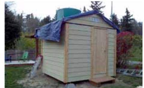
Waiting for a roof
