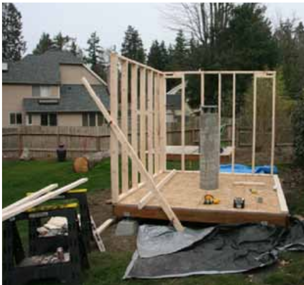
Pier with Floor and Wall Construction
